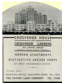
Constructed in 1935 by the Sassoon family, Grosvenor House stood as a distinguished Art Deco apartment building in Shanghai, representing one of the most prestigious residential addresses in the city. In the 1950s, the Van Roosbroek family established their residence within an apartment in this renowned building. 峻嶺寄廬乃1935年由沙遜家族建造，乃裝飾風藝術風格的建築，是彼時上海最為顯赫的公寓住宅之一。上世紀50年代，范·羅斯布魯克家族在此居住。
